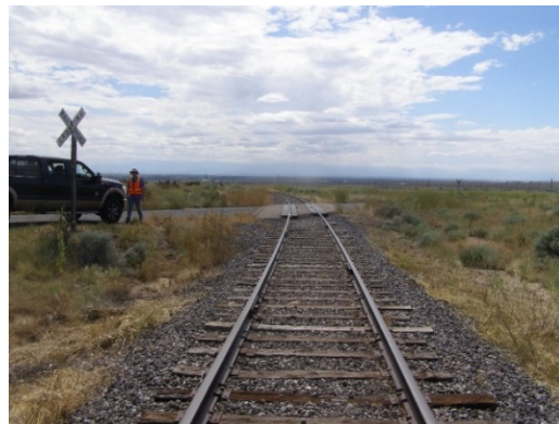
Main Track looking South at Junction Road At-Grade Crossing
