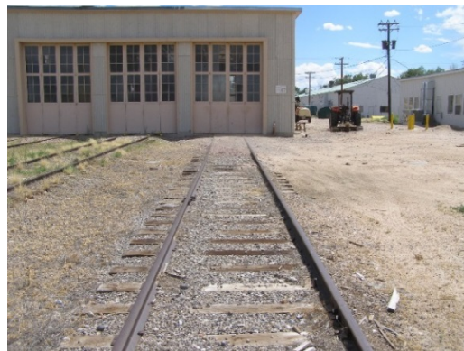
Locomotive Shop Track 3
