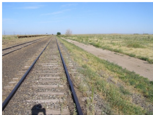
Classification Track 1 looking West
