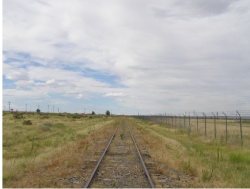
4 th Avenue Track looking North from 18 th
