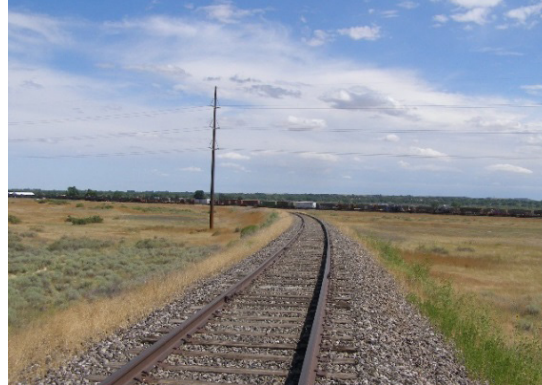
Main Track looking South along Eastern Mainline Wye Connection
