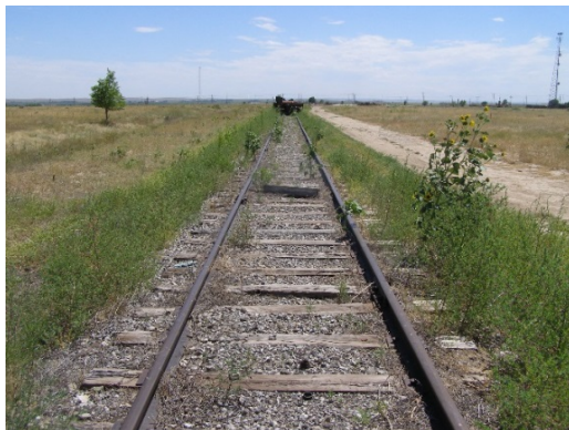
Track 113 South of 11 th St looking South
