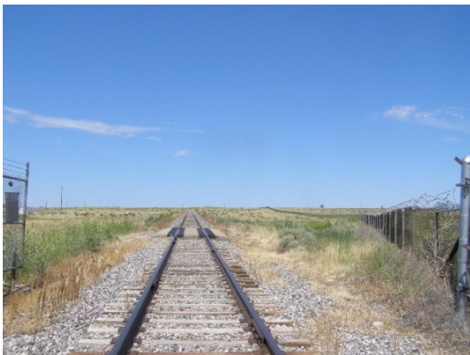
Main Track looking North from West Patrol Road Crossing
