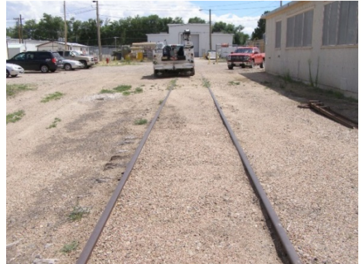
East Shop Track – Earthen filled
