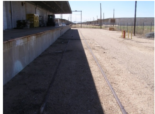
Paved Track 529 East end looking West
