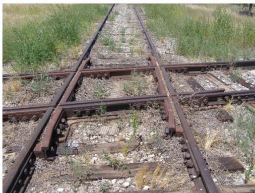
Diamond Crossing of Track 113 and 11 th St Track
