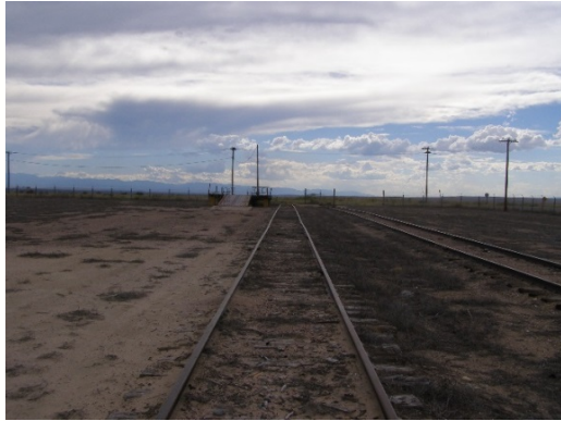
South Patrol Road Track Terminus, East of 1 st Arterial Rd West
