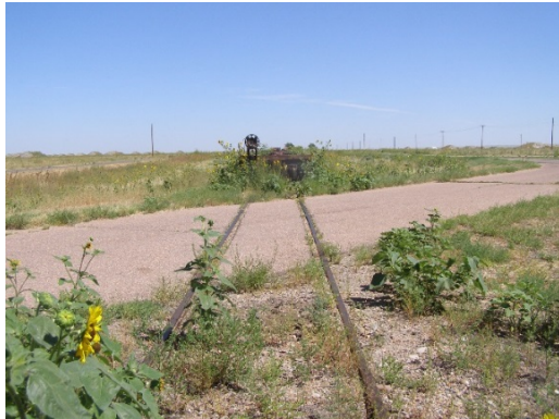
East Loop Track looking North near E-10 Street
