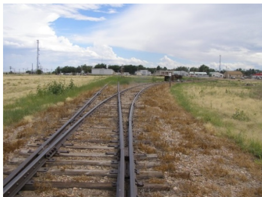
4 th Avenue Track looking South
