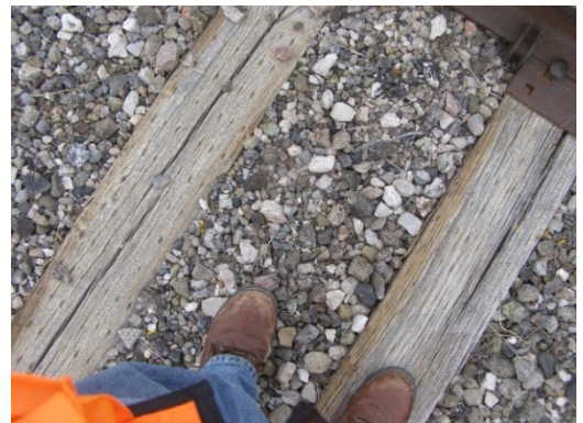
Main Track Ballast
