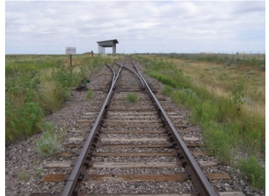
Main Track looking North from A-8 Street
