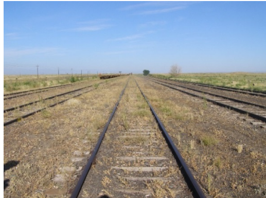
Classification Track 3 looking West
