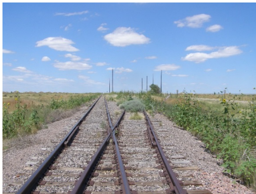
Main Track looking North from E-8 Street
