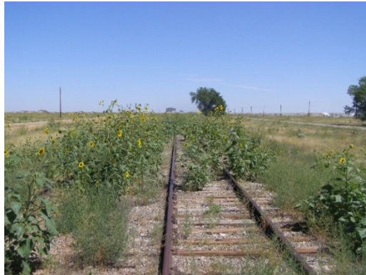
East Loop Track looking North near D-3 Street
