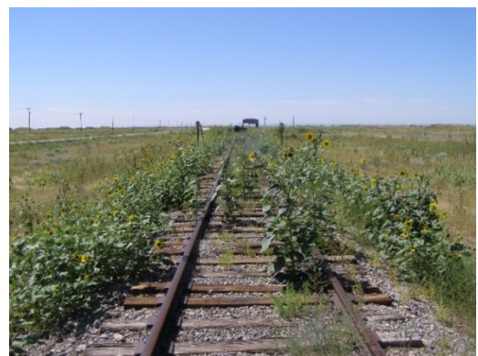
East Loop Track looking North near E-4 Street
