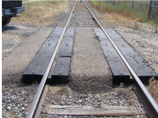
West Patrol Road Rubber Insert Crossing
