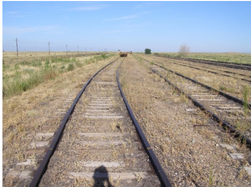
Classification Track 5 looking West
