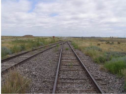
Main Track looking North from C-10 Street
