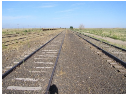
Classification Track 2 looking West
