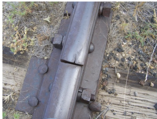
End Batter beginning of Split Head in Locomotive Tracks
