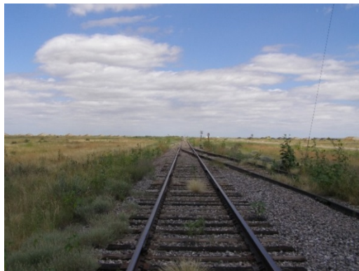
Main Track looking North from E-10 Street
