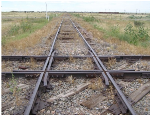
Diamond Crossing 4 th Avenue Track and South Patrol Rd Track
