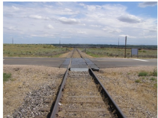
Main Track looking South at Main Entrance Road Crossing
