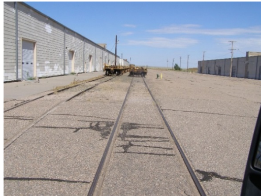
Warehouse Area 19 th St Track and Siding
