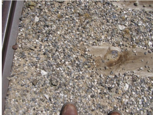
Track 3 Ballast – Gravel Sized
