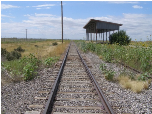
Main Track looking South from D-10 Street
