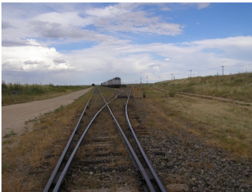
West End of Classification Yard looking North
