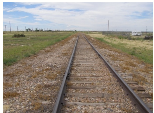
4 th Avenue Track looking North towards 11 th St
