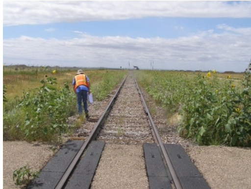
Main Track looking South from C-1 Street
