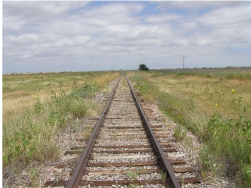
Main Track looking North from C-1 Street
