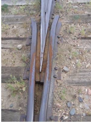
4 th Avenue Track (Locomotive Shop) Lead Track Frog
