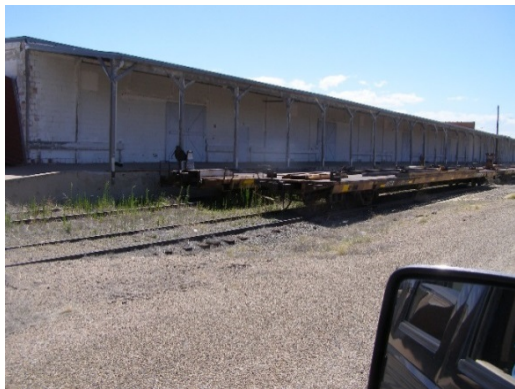
Track 529 and Siding Track near 17 th Ave
