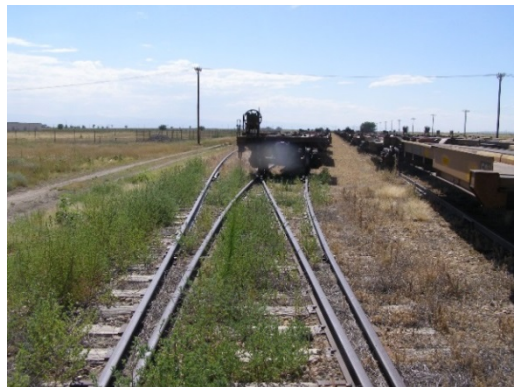
East Yard, South Track looking West
