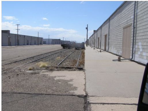
Warehouse Area 19 th St Track and Siding
