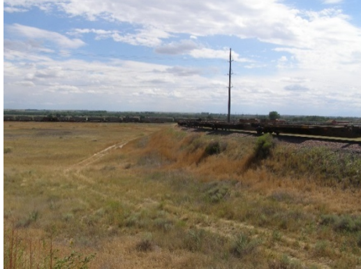
Main Track looking South at Western Mainline Wye Connection
