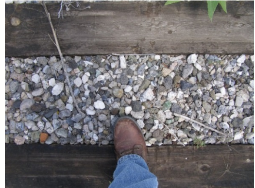
Main Track Ballast
