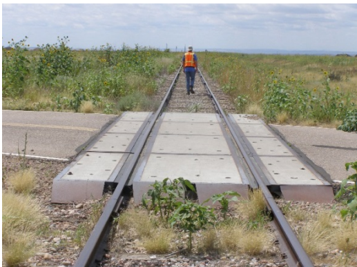
Main Track Concrete Crossing Panels at D-8/B-9 Street
