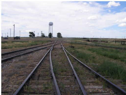
4 th Avenue Track looking North from Locomotive Shop
