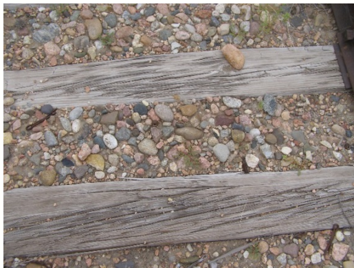
Well-graded, no-angular ballast
