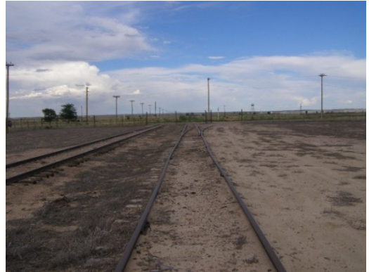
South Patrol Road Track looking East
