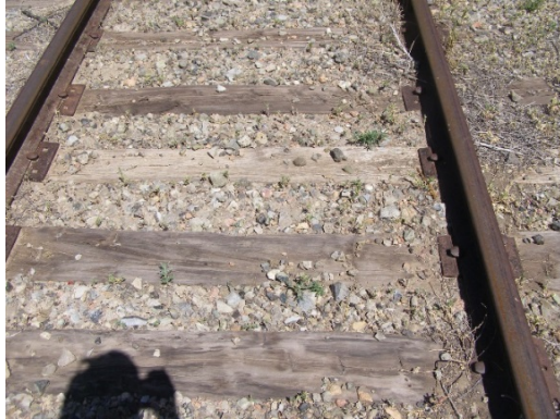
Warehouse Area Ballasted Track
