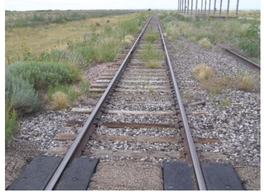
Main Track looking South from C-10 Street
