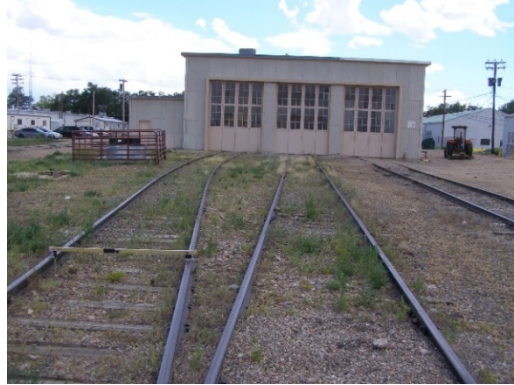
Locomotive Shop Tracks
