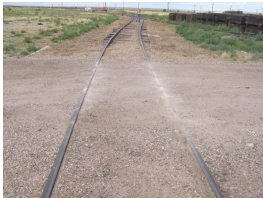
4 th Avenue Track Earthen At-Grade Crossing
