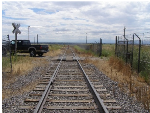
Main Track looking South from West Patrol Road Crossing
