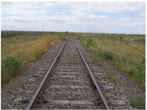
Main Track looking South from A-8 Street
